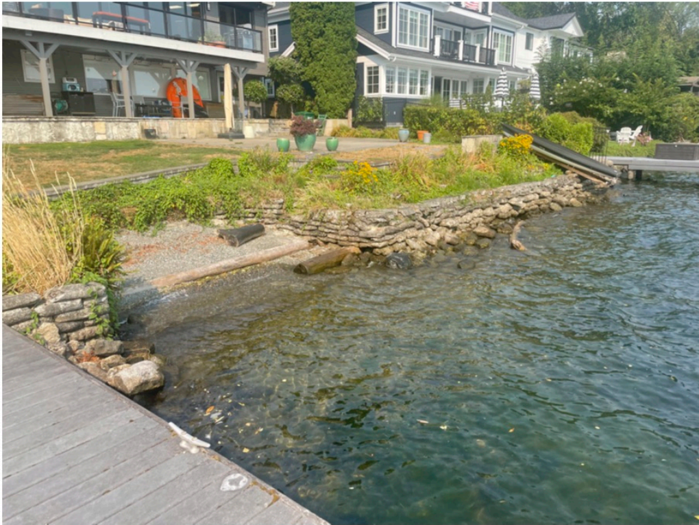
Photo 3 - Existing shoreline conditions north of dock showing cove and bulkhead.
